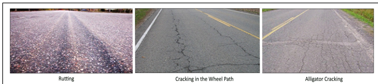
Figure 4: Structural distresses
