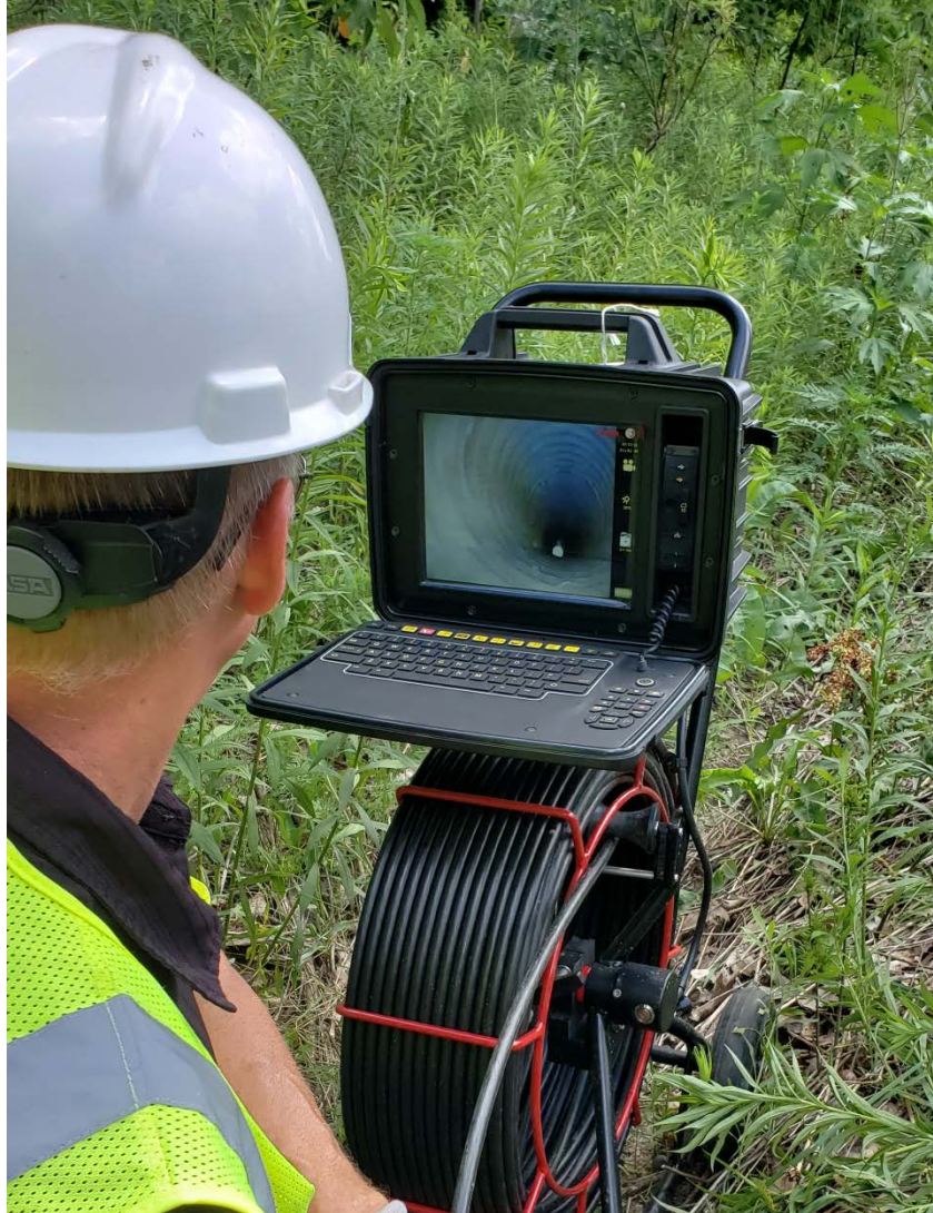
Figure 6-4: The Road Commission for Kalamazoo County used a sewer camera to inspect some culverts
