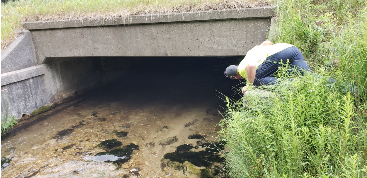
Figure 4-1: Antrim CRC inspecting a concrete box culvert
