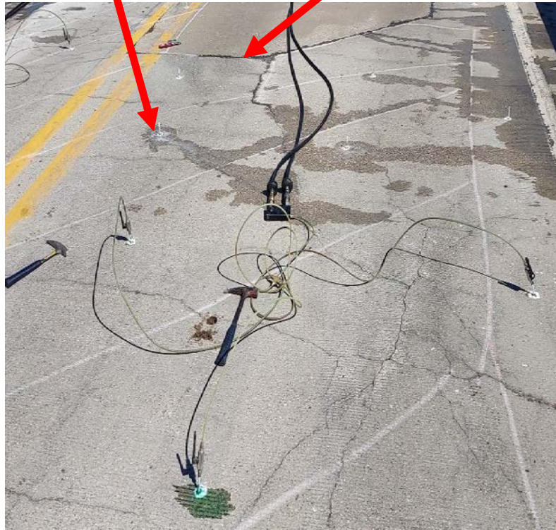
Epoxy Injection Process
