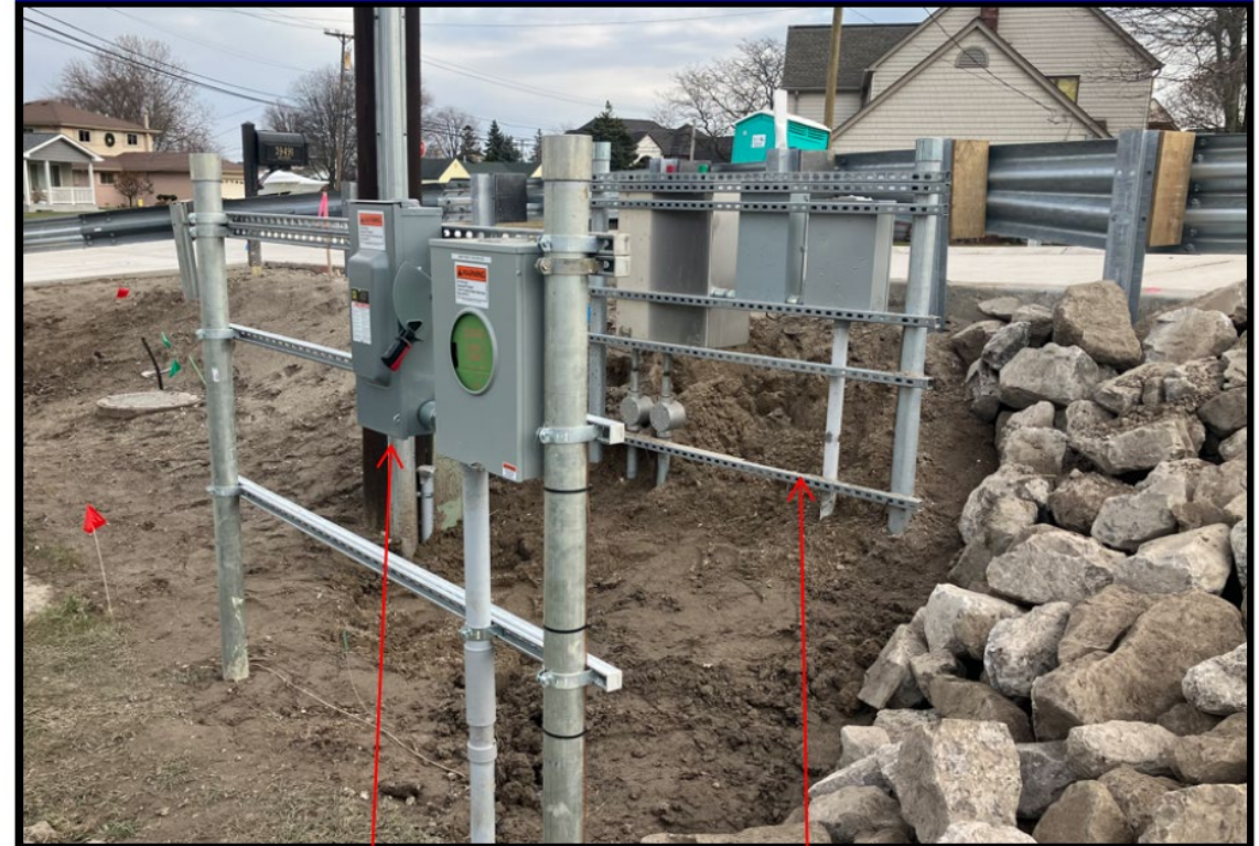
West Archer Drive: Pump Station Racks during construction
