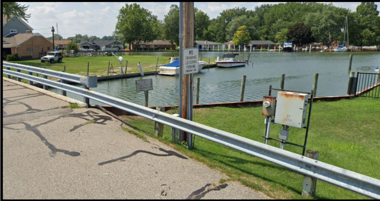
West Archer Drive: Pump Station Rack when Surveyed
