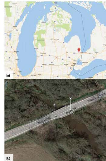
Fig. 1: Bridge repair site: (a) location in Michigan, and (b) aerial view
