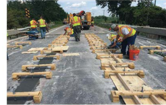
Figure 7. Photo. Installation of UHPC connection repair project on the Kilgore Road Bridge over Pine River in Kenockee Township, MI.
